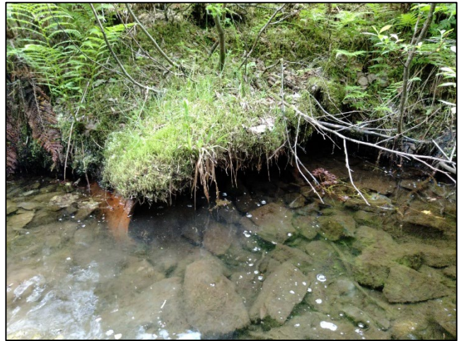
Figure 3.– Outlet of culvert at waypoint 479.
